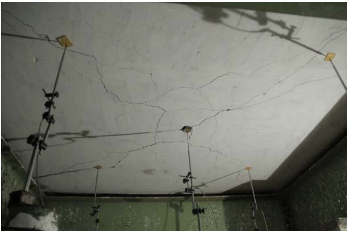
Figure 3.57 – Observed Crack Pattern of Slab Specimen TF-CV-1
