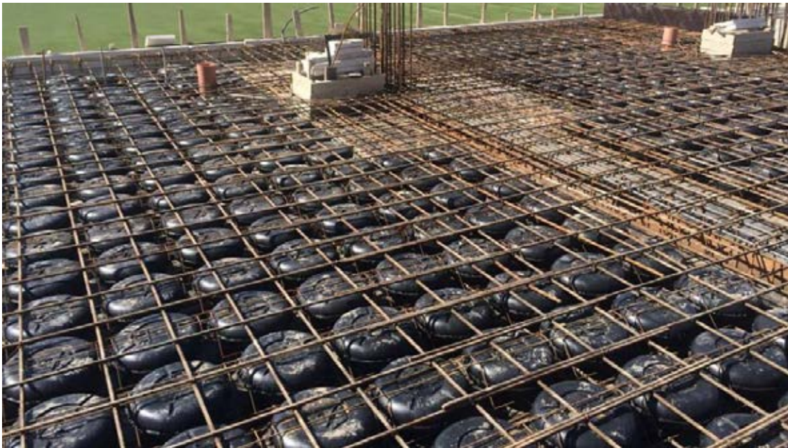
Figure 1.8 – Two-way Voided Slab with Plastic Void Formers (Source: www.cobias.com)
