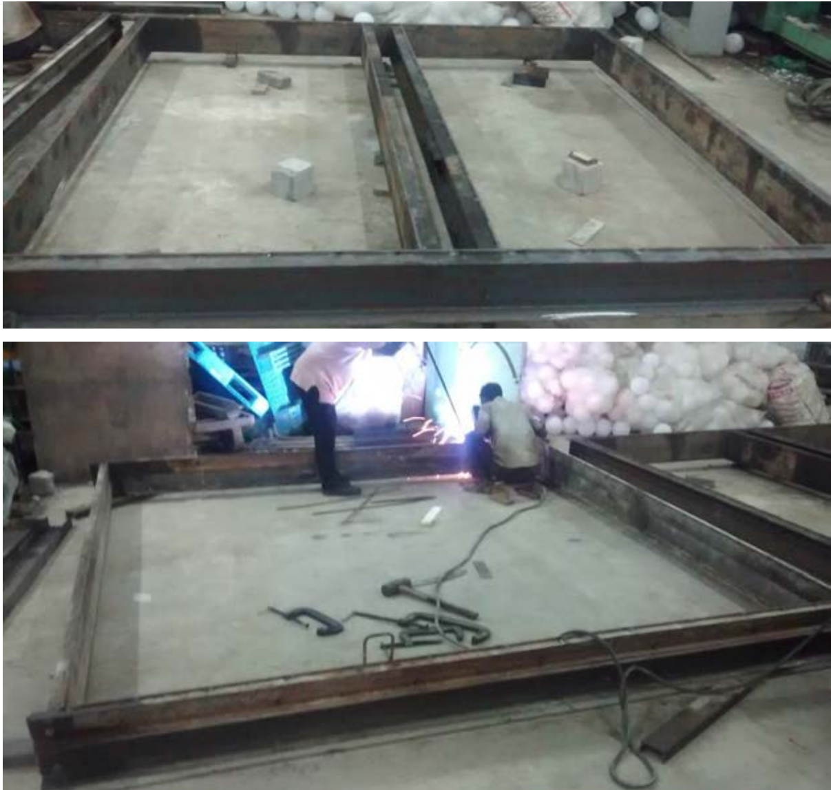
Figure 3.12 – Fabrication of Steel Mould in Progress
