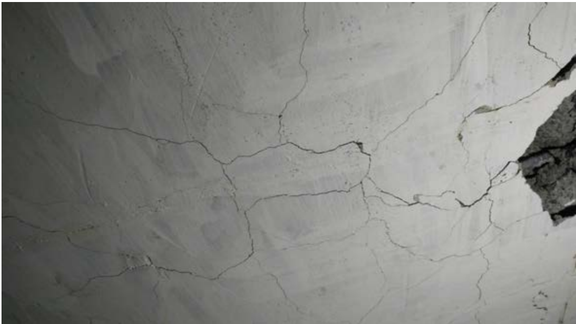
Figure 4.35 – Observed Crack Pattern of Slab Specimen V6
