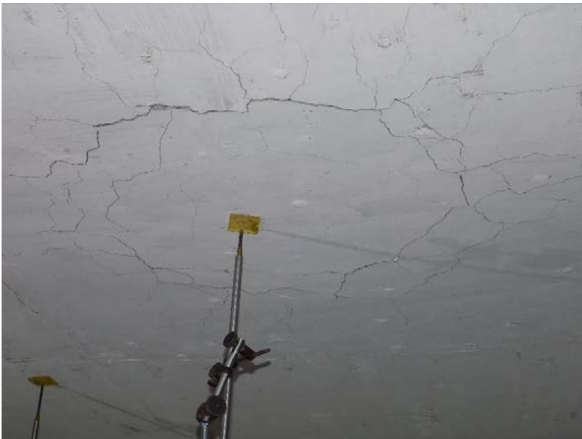
Figure 4.29 – Observed Crack Pattern of Slab Specimen S
