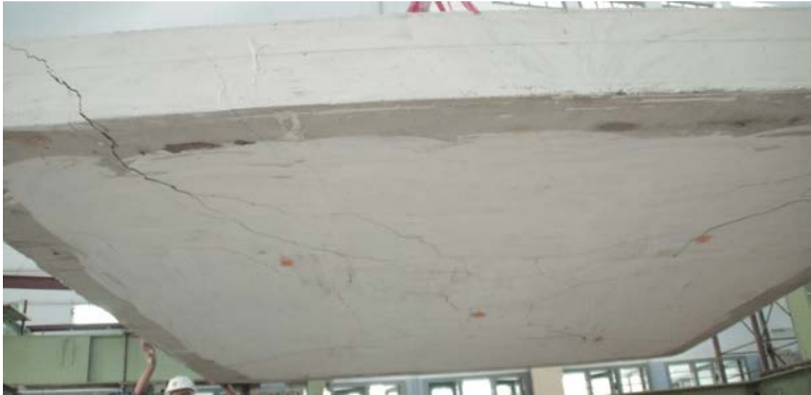
Figure 3.58 – Observed Crack Pattern of Slab Specimen TF-CV-2
