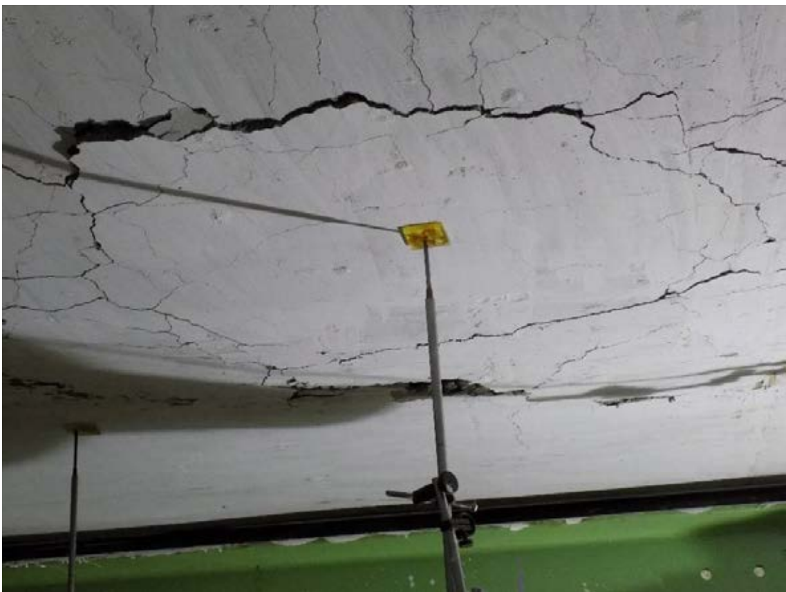
Figure 4.31 – Observed Crack Pattern of Slab Specimen V2
