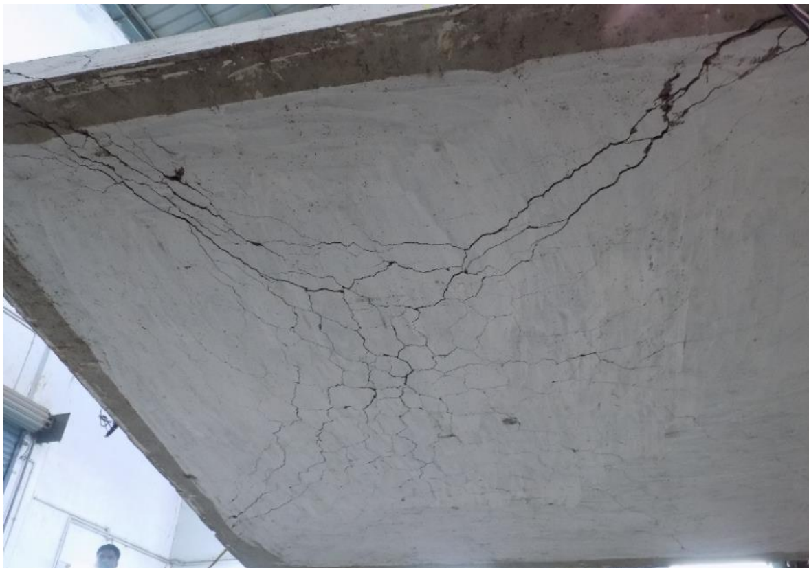
Figure 3.55 – Observed Crack Pattern of Slab Specimen TF-Solid
