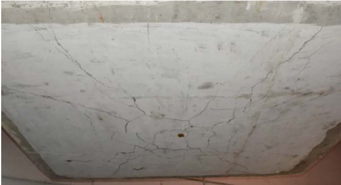
Figure 3.56 – Observed Crack Pattern of Slab Specimen TF-S180V
