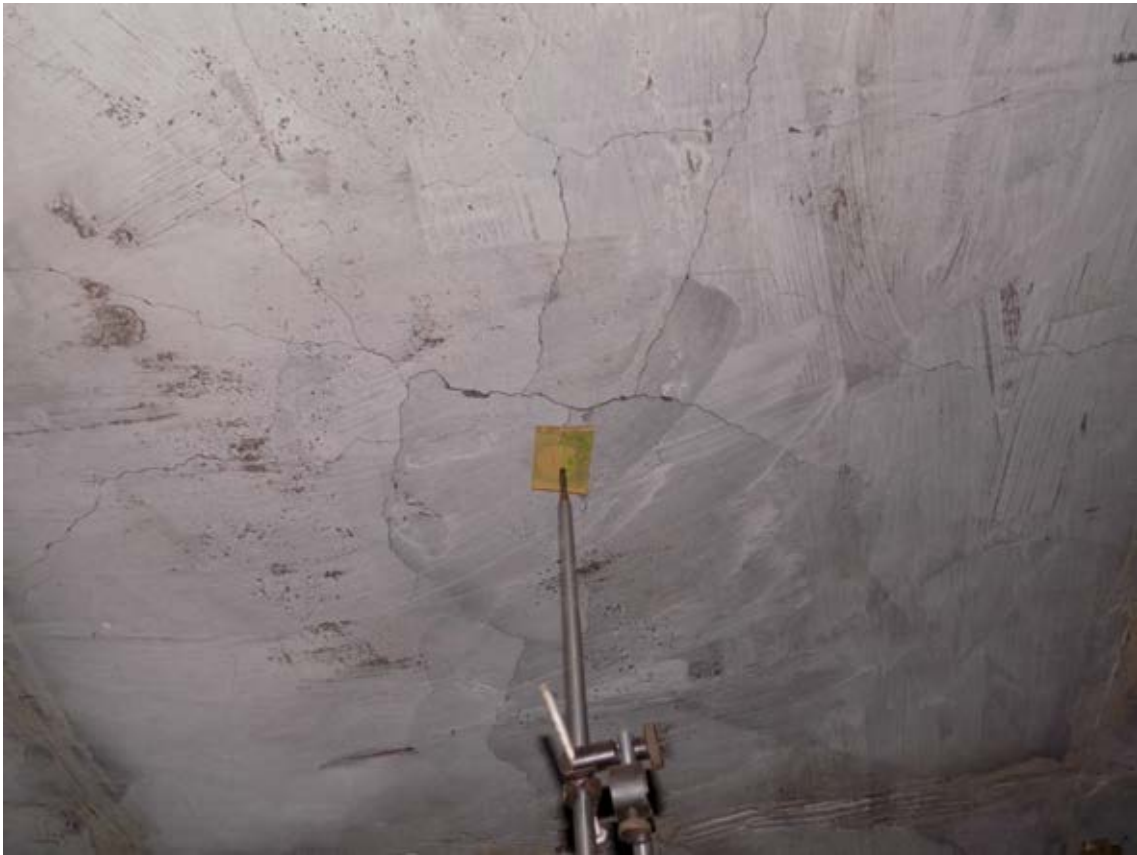
Figure 4.34 – Observed Crack Pattern of Slab Specimen V5
