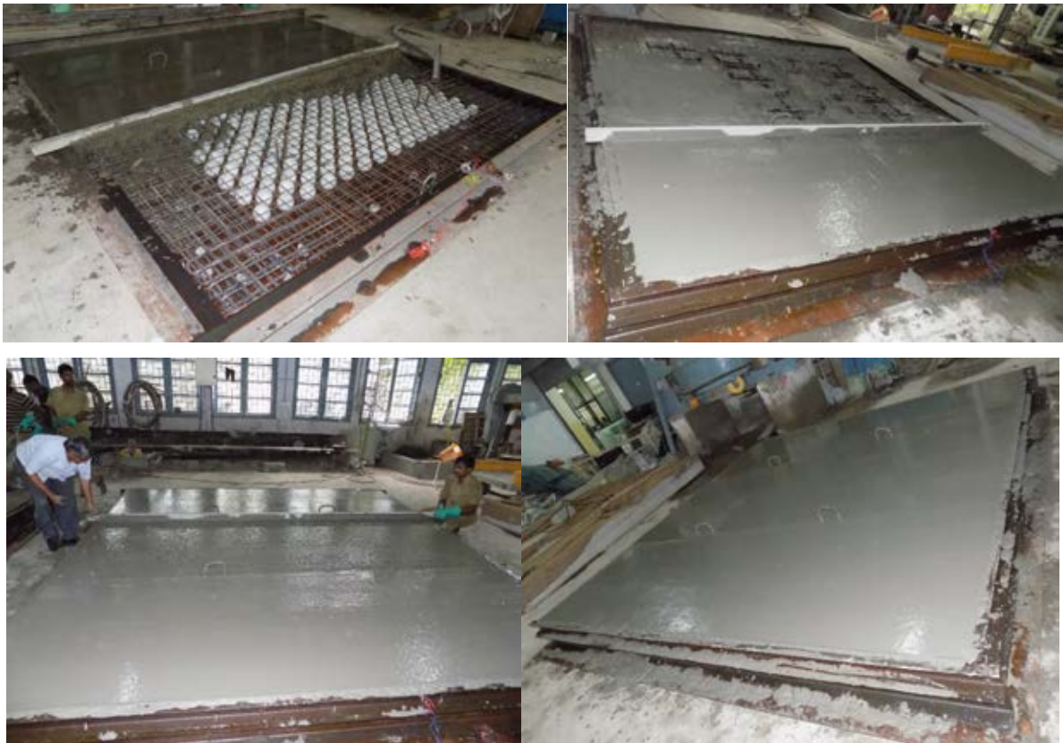
Figure 3.19 – Concreting in Progress
