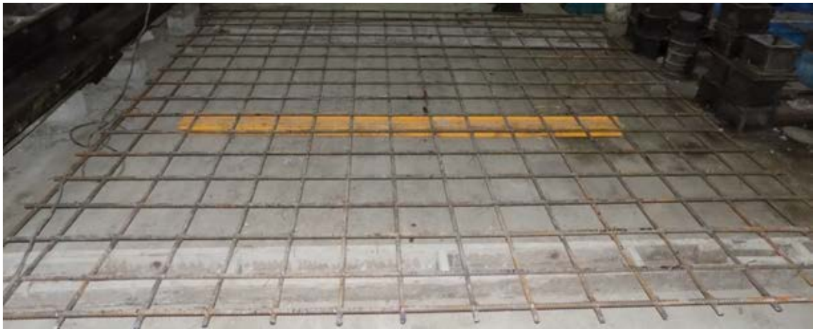
Figure 3.13 – Typical Reinforcement Mesh
