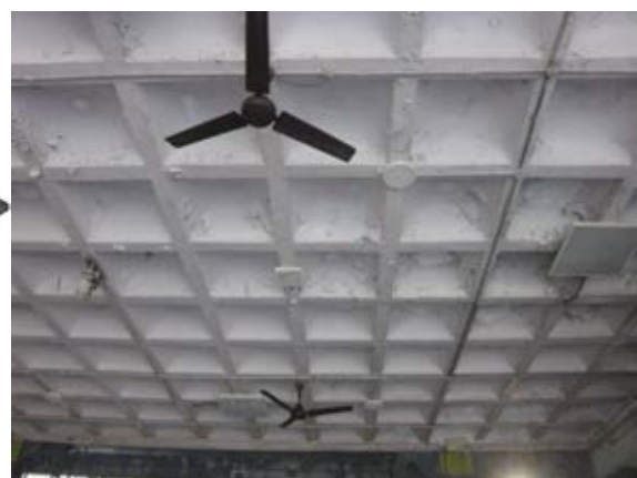
(b) Two-way Slab (Waffle Slab)
