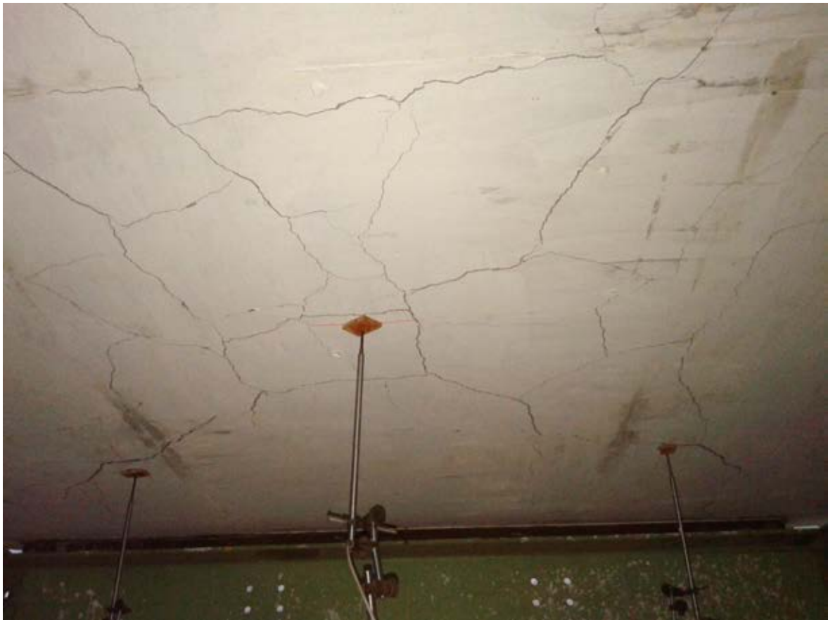
Figure 3.59 – Observed Crack Pattern of Slab Specimen TF-CV-3
