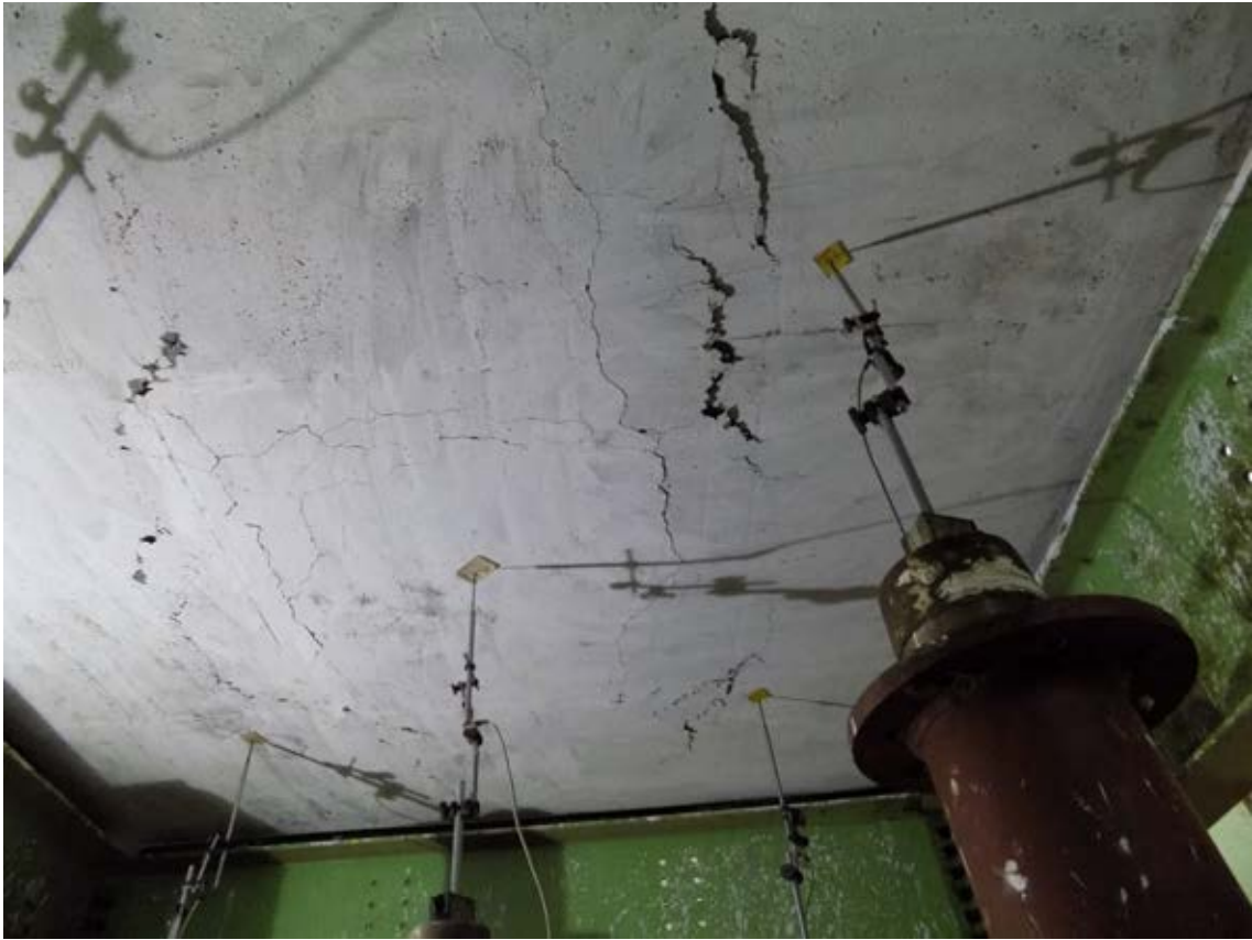
Figure 4.32 – Observed Crack Pattern of Slab Specimen V3
