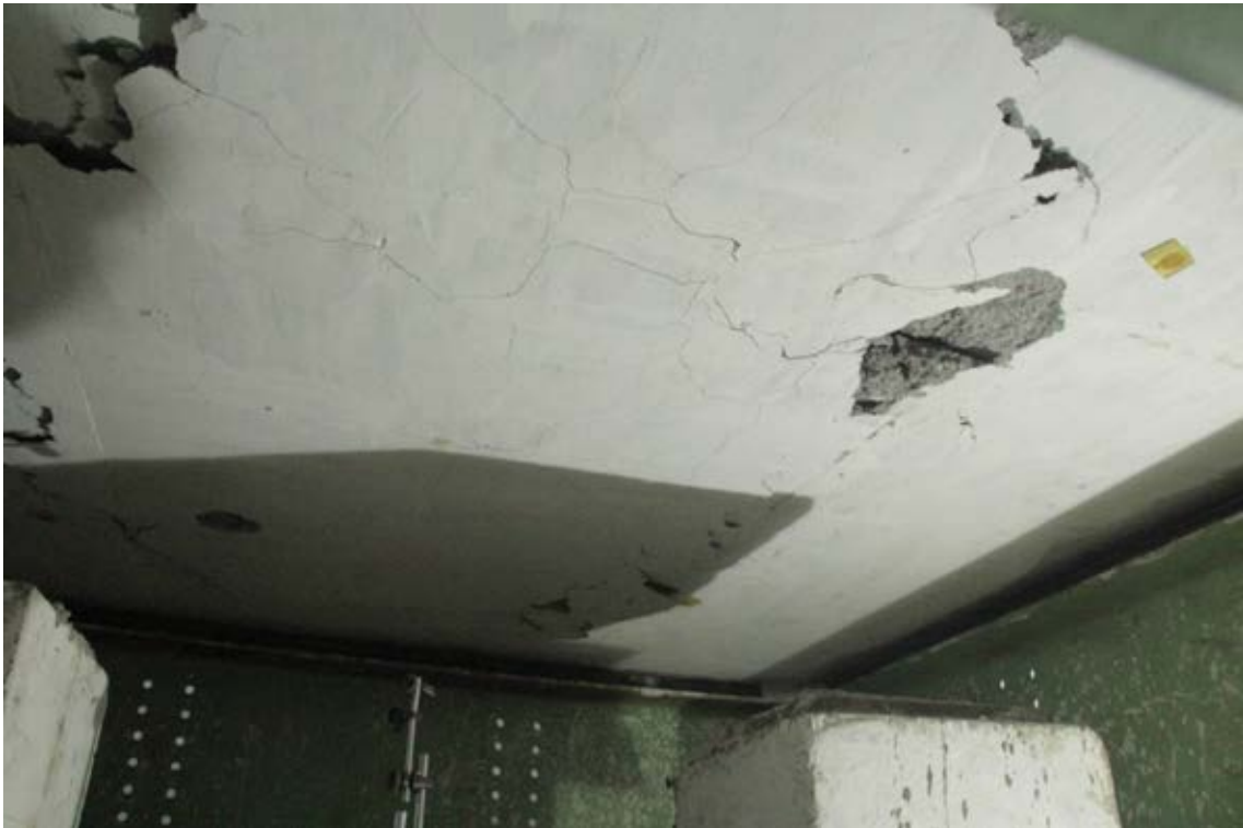
Figure 4.36 – Observed Crack Pattern of Slab Specimen V7
