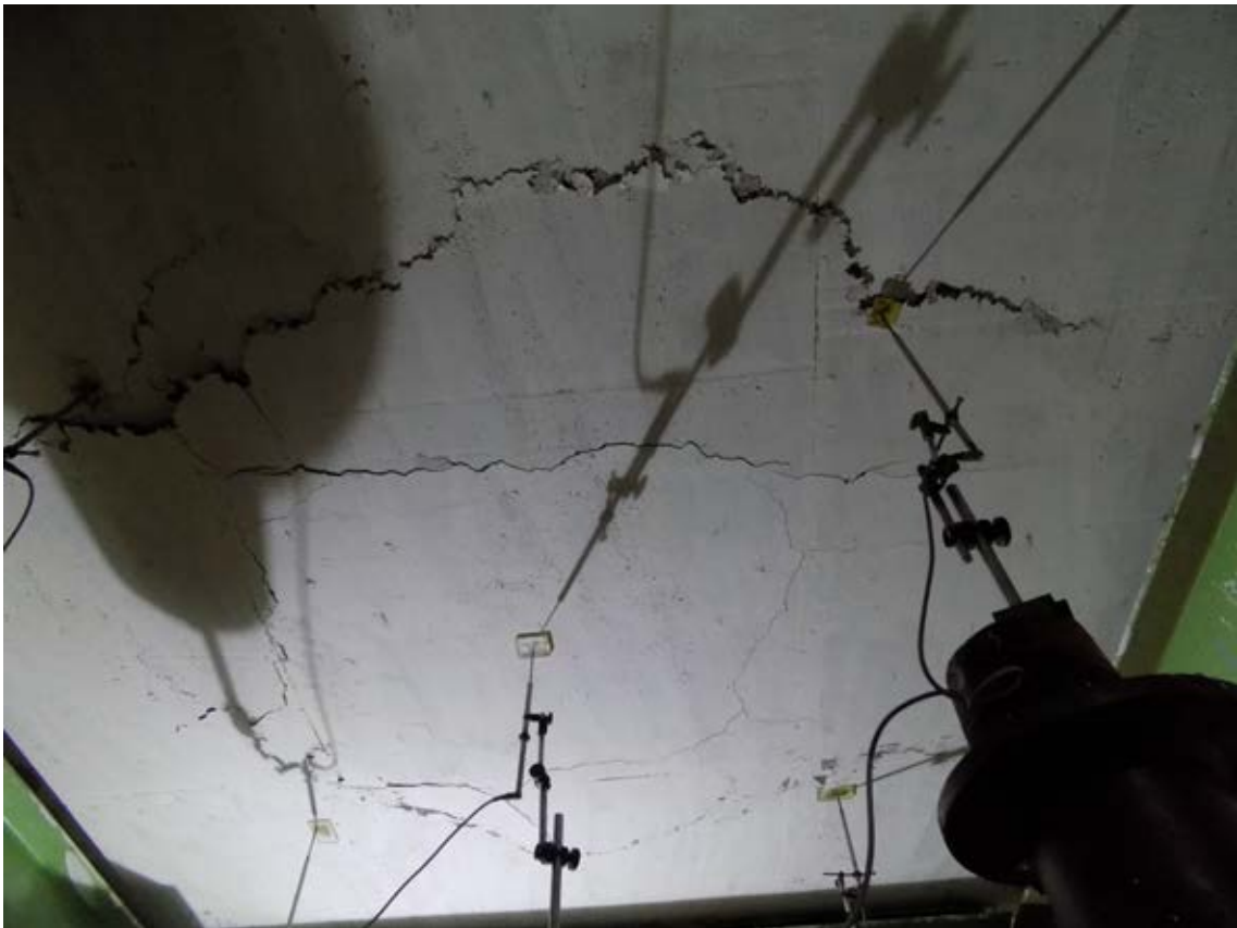
Figure 4.33 – Observed Crack Pattern of Slab Specimen V4
